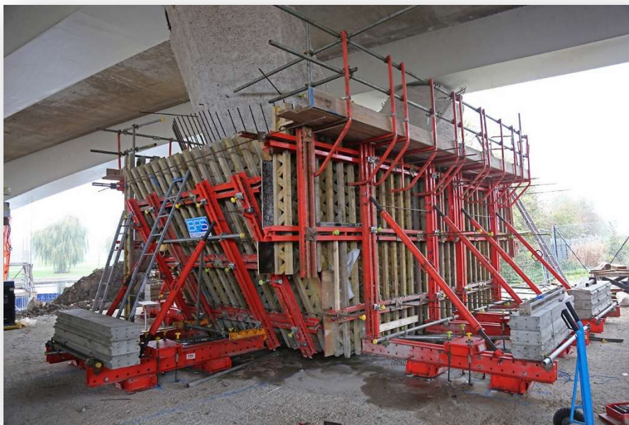
Construction of Concrete Jacket on Nene Bridge Piers
